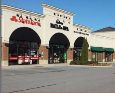
Arbor Crossing Madison, Alabama 35756
